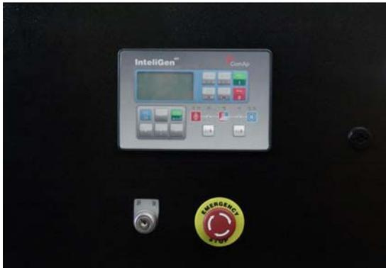
**Automatic Parallel Control Panel** This new automatic parallel system adopts intelligent modules, inserted and folded installed, no need the peripheral relay and logic circuit. The main switch adopts electronic breaker or frame breaker, combined together with the generator, which is very reliable. One generator, one panel. The panel can be used both for singly and parallel. It is only need to parallel generator with such panel when the capability needs to be enlarged in the future.
