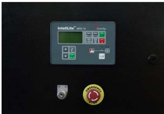
**Auto Module Control Panel** is the configuration for nobody on duty controlling generators. This kind of panel adopts auto module control system, with large LCD display to show the menu.
